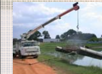
Aerator mechanical and electrical repair
