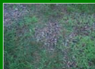
Completed well decommissioning
