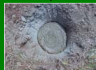
Concrete layer placed over casing filled with bentonite
