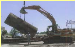
A UST Removal that took place in Fort Wayne, Indiana
