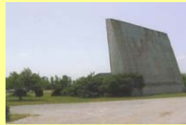
Property in Muncie, Indiana that Creek Run completed a Phase I Environmental Property Assessment
